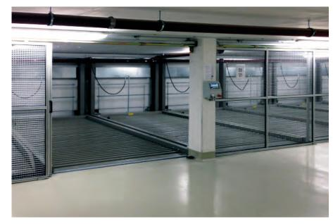
Metal gates are included in the scope of delivery of your semi-automatic system. Optionally you can also choose other types of gate coverings.
