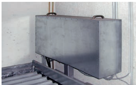
Sound insulation hood for the power unit
